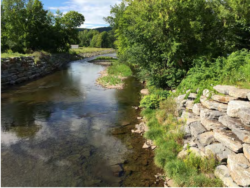
Photo Source: Milone & MacBroom, Inc. (2015)
