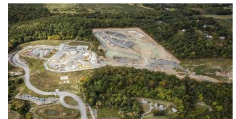
Figure 9.2 Aerial view of the Shaft 5B site.
