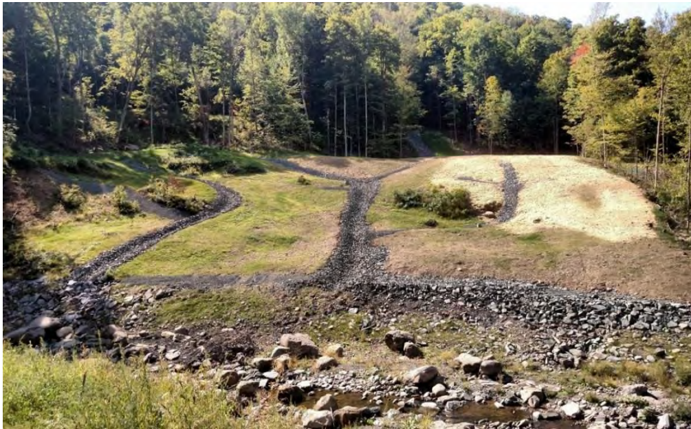
Figure 4.18 Wright Road site after construction.
