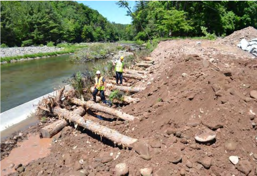
Figure 4.23 Installing root wad revetment.
