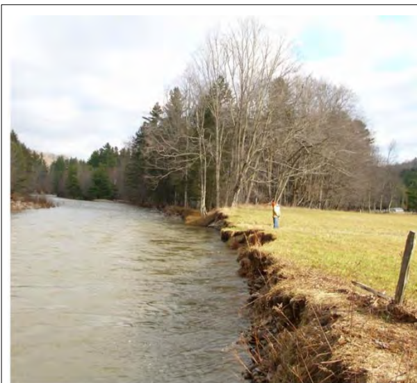
Figure 4.22 Eroding streambank before bioengineering treatment.
