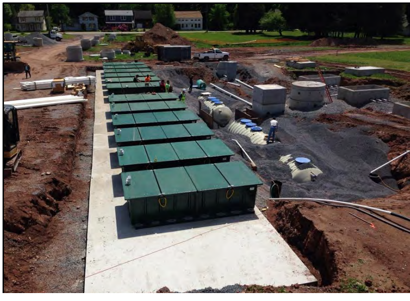
Figure 3.1 Installation of Orenco treatment units in Lexington.
