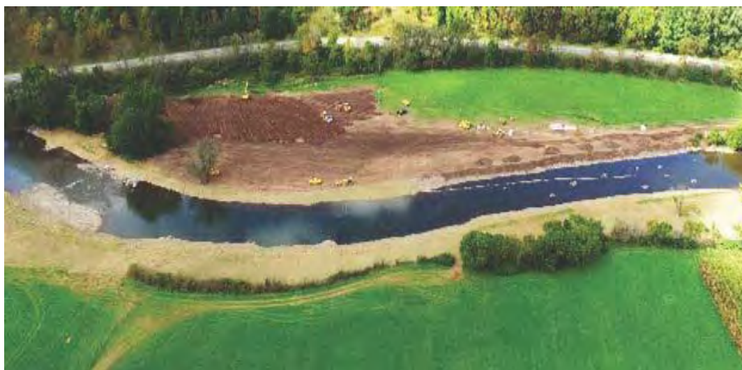
Figure 4.20 More property after construction.
