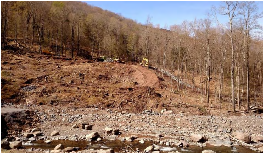
Figure 4.17 Wright Road hillslope before construction.
