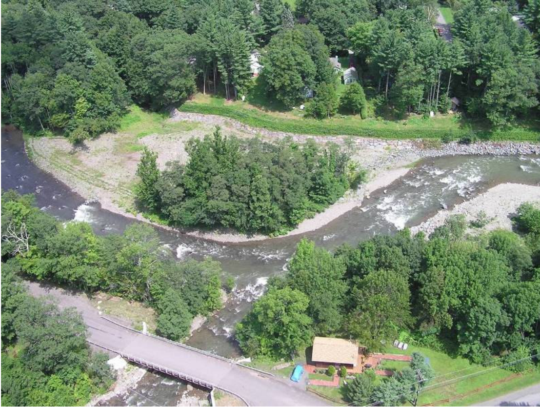
Figure 3.3. Esopus Creek at Woodland Valley Restoration Demonstration Project. The photo was taken one year after completion.
